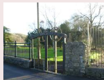
Sluice gate at Chewton Keynsham
