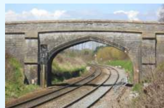
Footbridge over Brunel's railway
