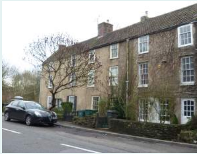
Former Hat factory
