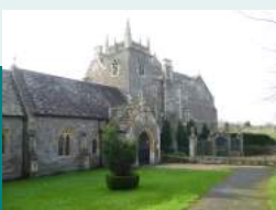
Hanham Court and Church
