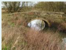
Londonderry Wharf- bridge
