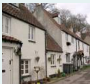
Hanham Mill cottages
