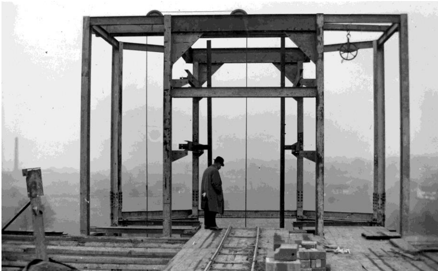
Part of the girder construction 1922
