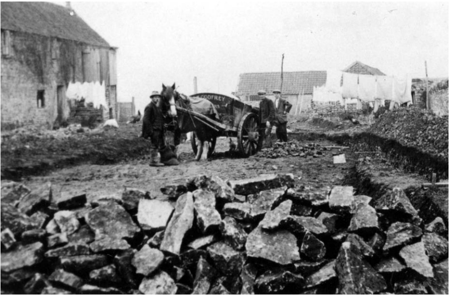
Clearing the site
