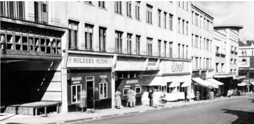
The Union Street shops were repaired but small 'utility' windows had to be fitted, as a temporary measure.
