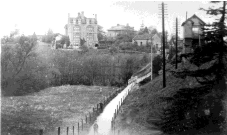
Fig. 6 – The footbridge over the Chew
