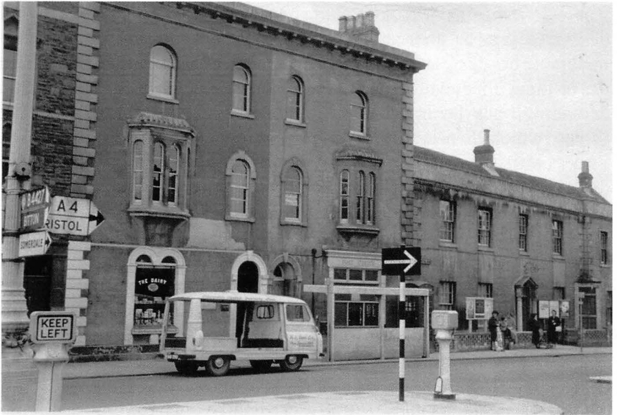
Figure 9. West End dairy with Exon's delivery van outside
